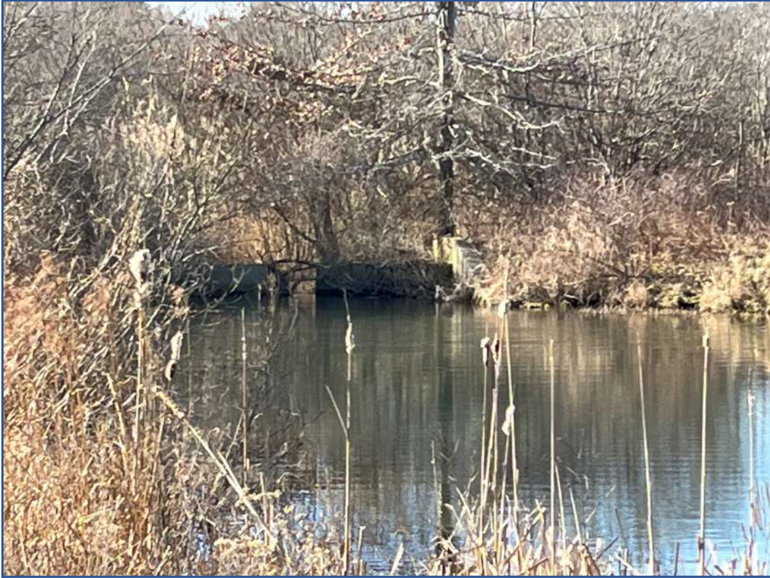
Concrete spillway at the southwest corner of the detention pond
