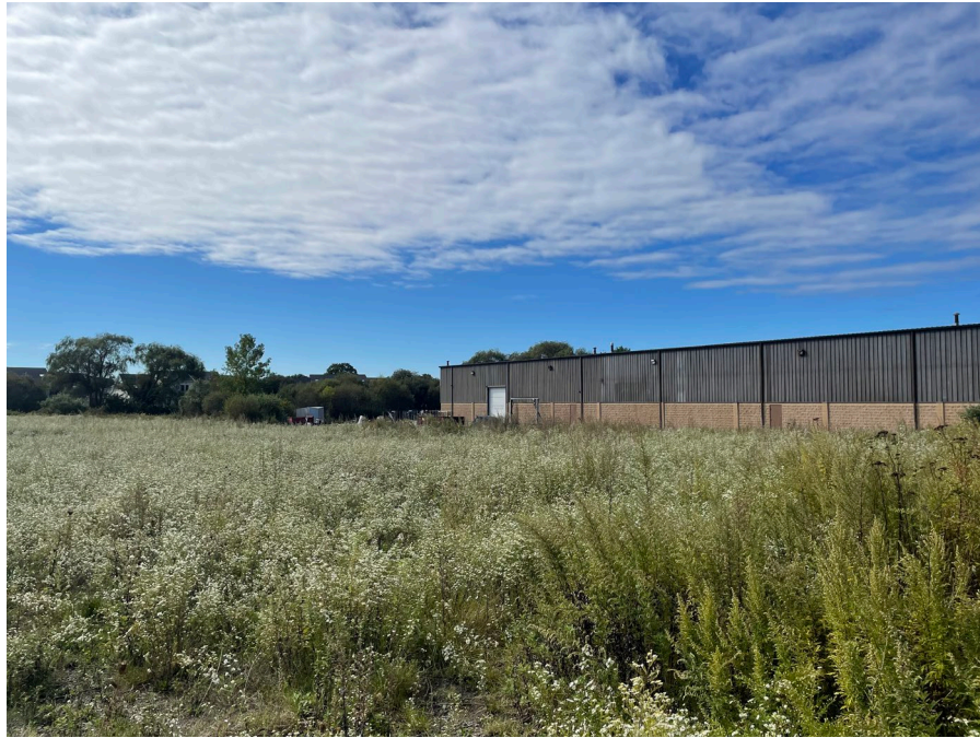
Photo 3: View of the existing warehouse facing southwest from near the end of the access drive.
