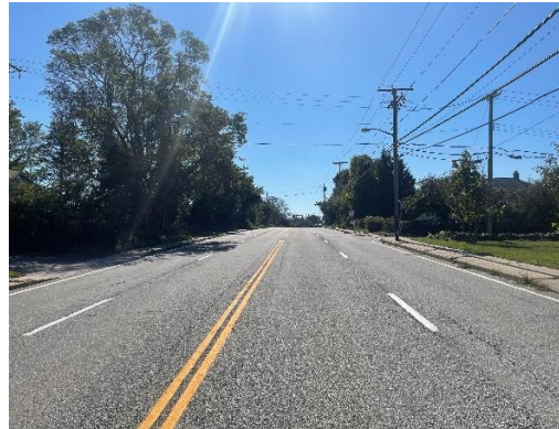
Photo 1: West Main Road.
