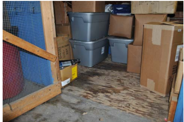
Storage shed interior at upper field
