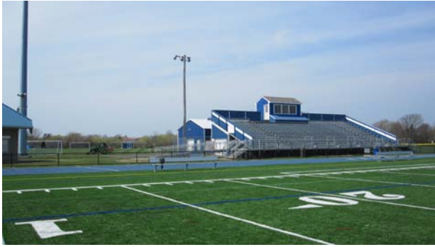
New bleachers and storage facility
