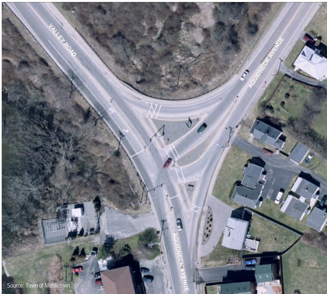
Figure 9. Valley Road at Aquidneck Avenue
