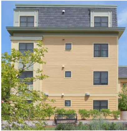
Fiber-cement horizontal lap siding, smooth side with varied width exposures
