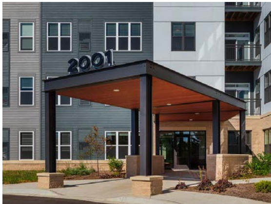
Painted steel frame porches with wood & stainless-steel cable handrails
