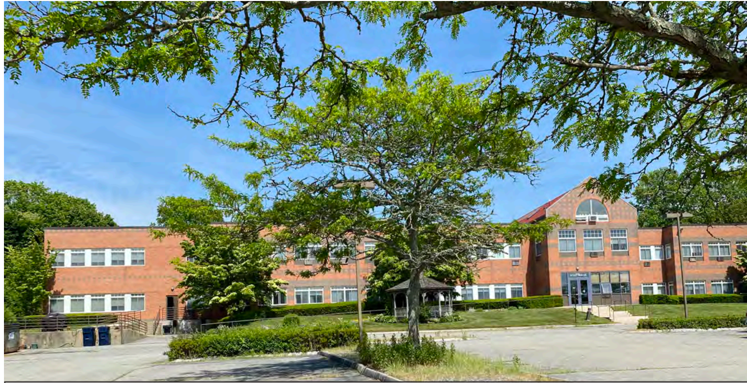
Existing West elevation of West House I. Proposed connection to West House II at building bumpout.
