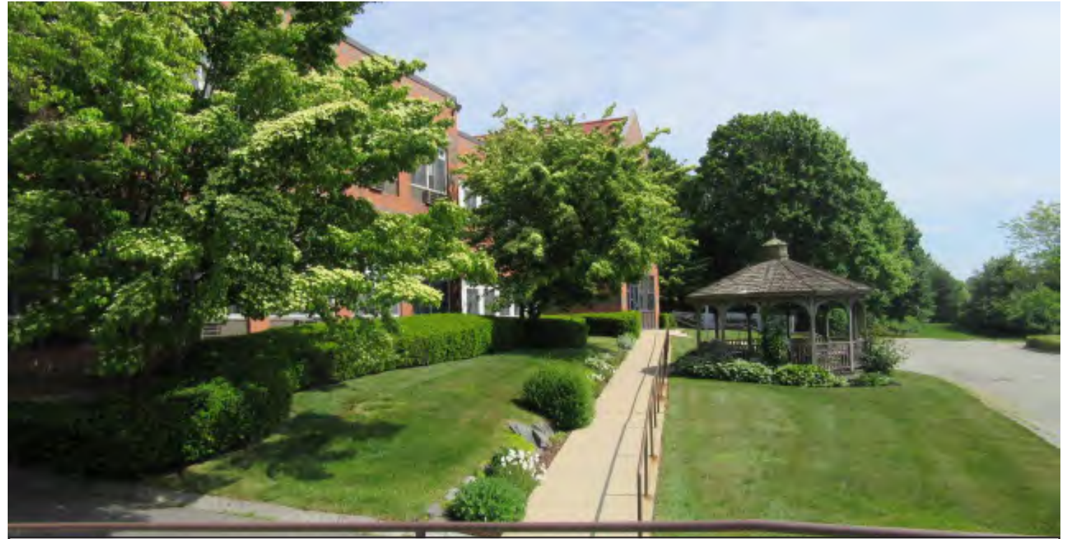
Existing ramp from Northwest corner of West House I up to proposed connection at West House II.
