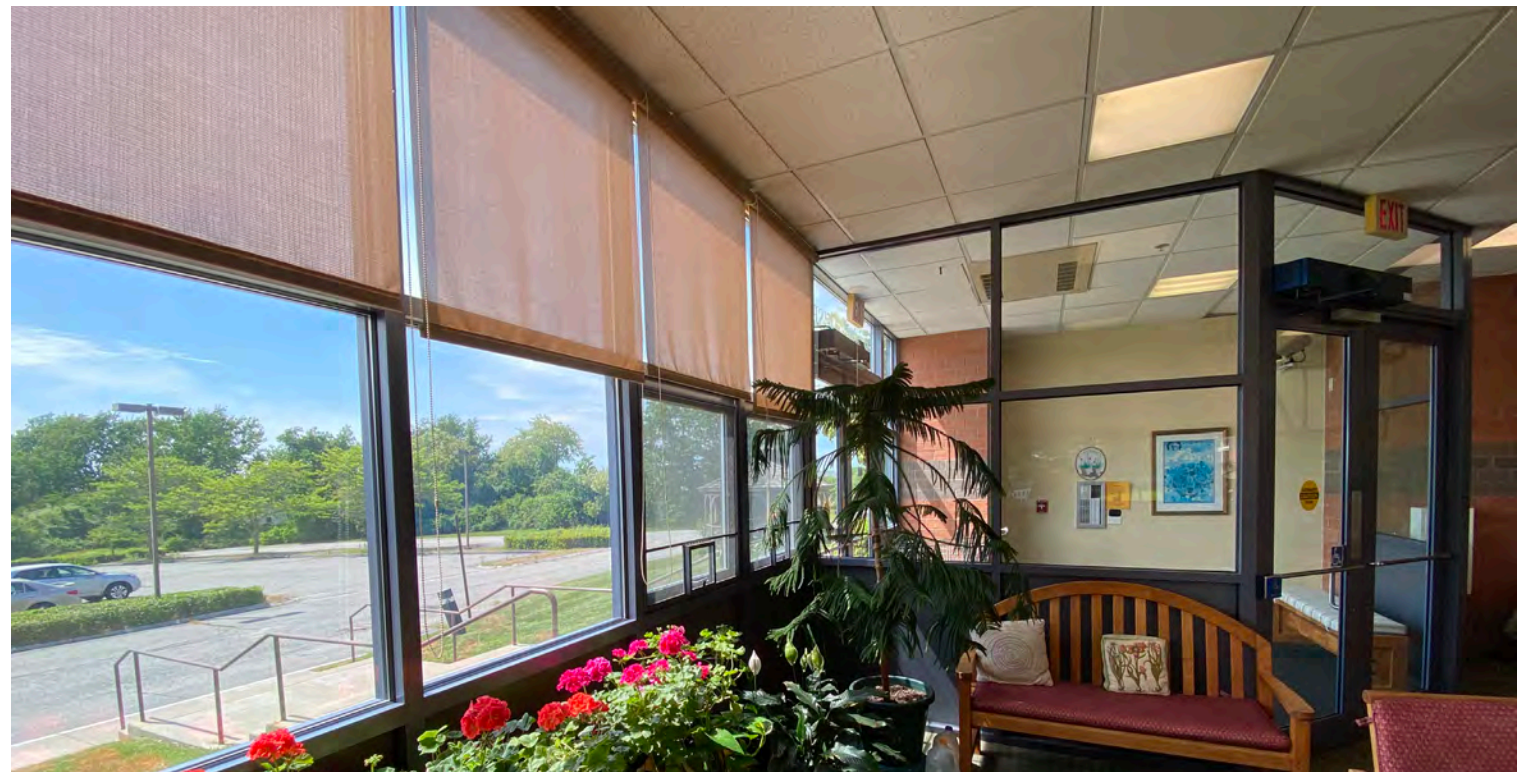
Existing solarium at West House I, where connection to new building is proposed.
