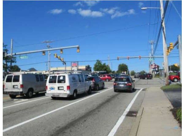
East Main Rd facing NB toward Valley Rd
