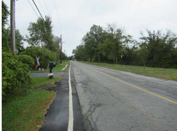
Paradise Ave facing south
