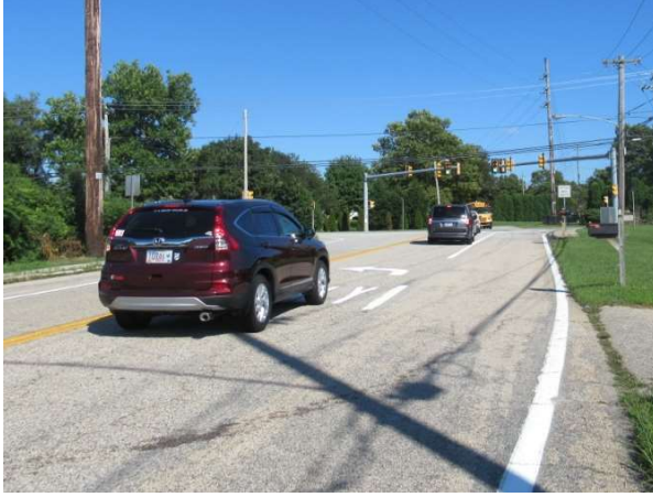
Greene Ln facing EB toward West Main Rd
