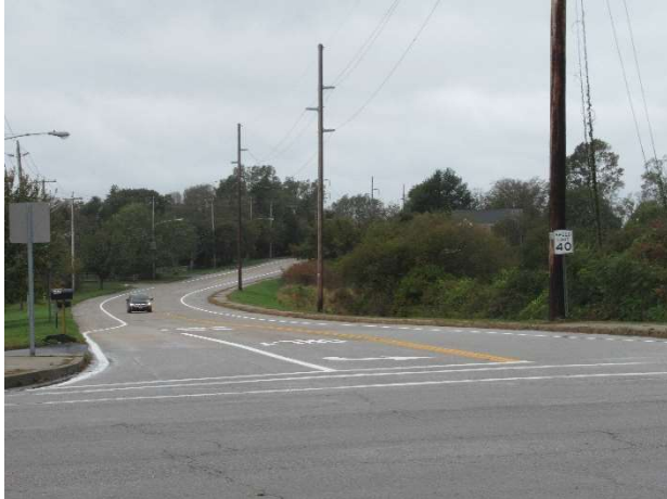
Facing west toward Greene Lane at West Main Rd
