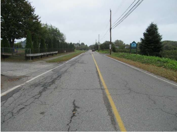
Third Beach Rd facing south
