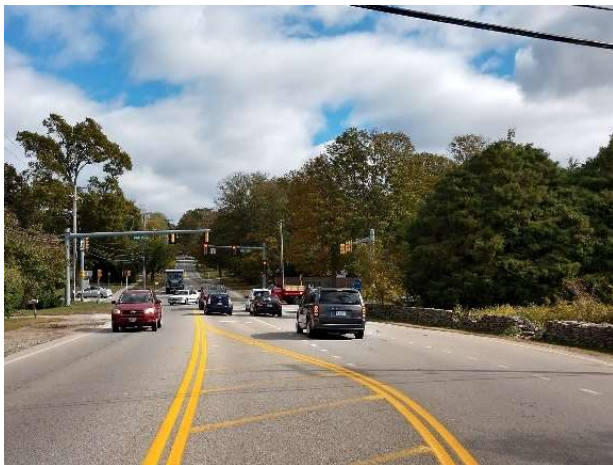
Green End Ave facing east toward Valley Rd
