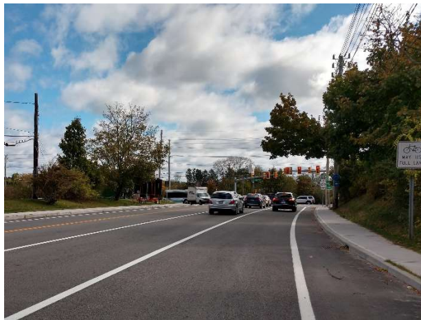
Coddington Hwy facing east toward W. Main Rd
