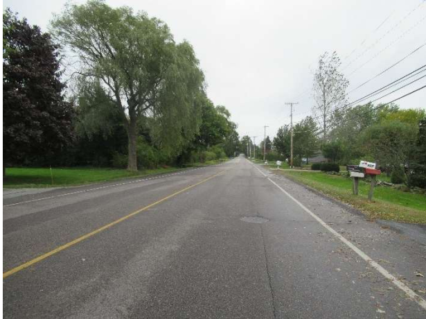
Green End Ave facing east
