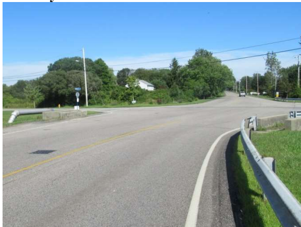
Green End Ave facing EB toward Berkeley Ave/Paradise Ave
