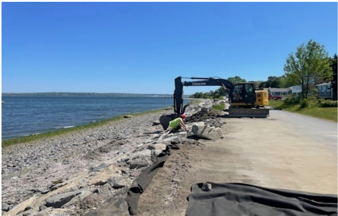
Prudence Island, Portsmouth seawall restoration (2024).
