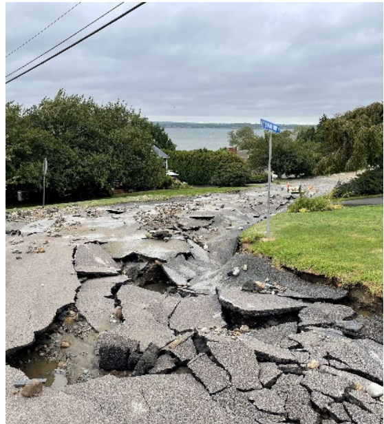
Underground catch basin (left) and road (right) collapsed after heavy rainfall from the remnants of Hurricane Ida in 2021. Photo credit: Portsmouth Police Department.
