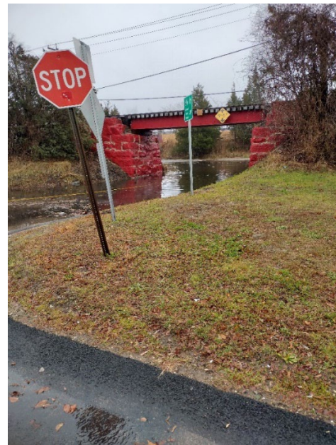
Road flooding at the entrance to Common Fence Point, Portsmouth. Grant money was used to install a better drainage system to reduce the flooding depicted above, but concerns grow as tides creep higher and water egresses in from the drainage system during extreme high-tide events.
