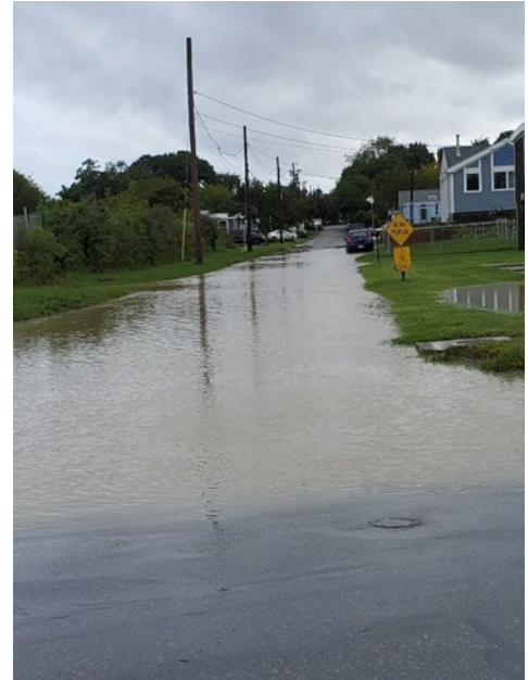
Flooding in Portsmouth.
