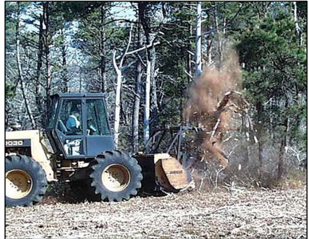
Figure 29: Front end loader with Fecon mastication head Credit: William Patterson III, funded by Joint Fire Science Exchange
