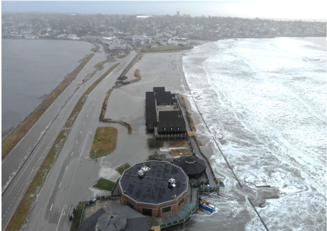
Easton Pond Dam South (left) and Easton's Beach (right) during a storm in December 2023. Photo credit: City of Newport.
