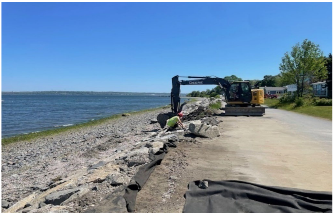
Prudence Island, Portsmouth seawall restoration (2024).
