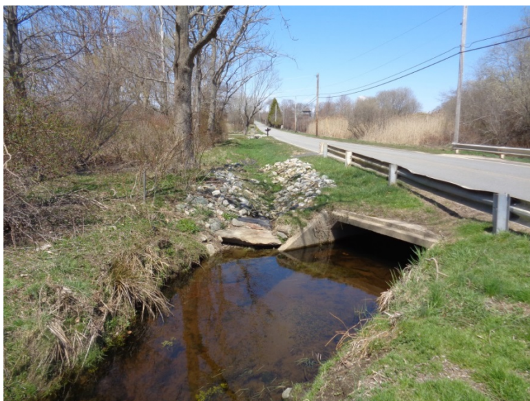
Berkeley Avenue Maidford River Crossing
