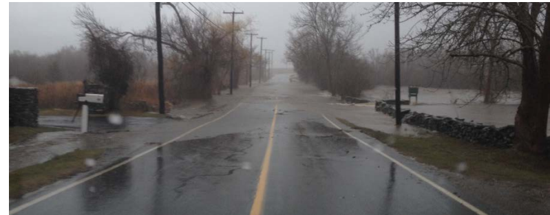
Roadway flooding is an ongoing problem in portions of the Maidford River watershed.
