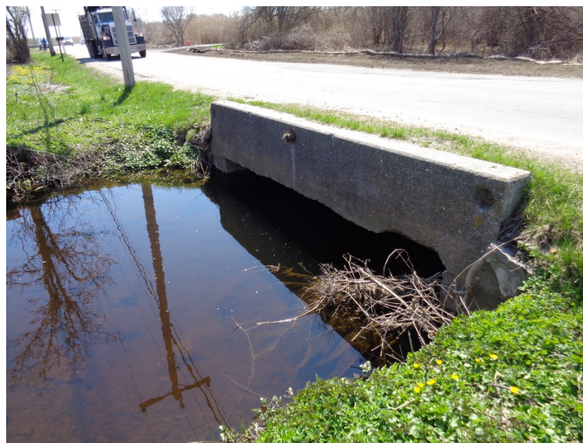
Paradise Avenue Maidford River Crossing
