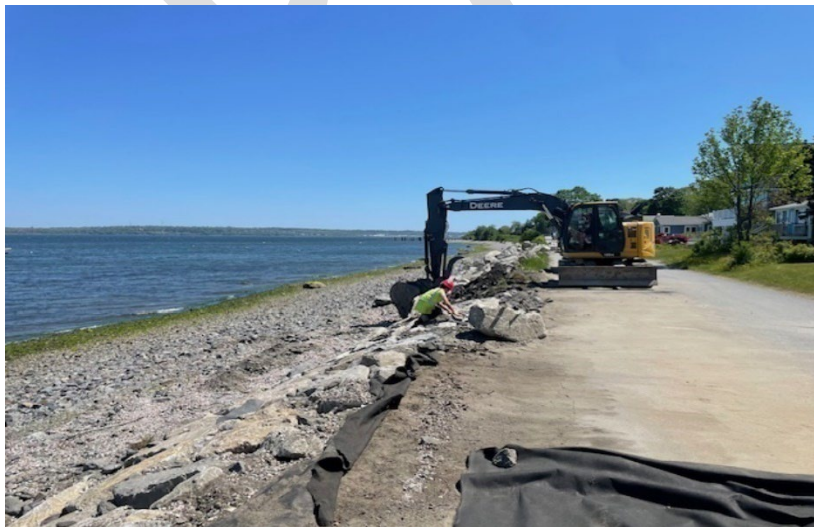
Prudence Island, Portsmouth seawall restoration (2024).
