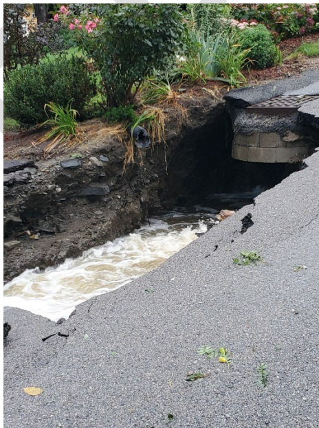
Road (above) and underground catch basin (left) collapsed after heavy rainfall from the remnants of Hurricane Ida in 2021.
