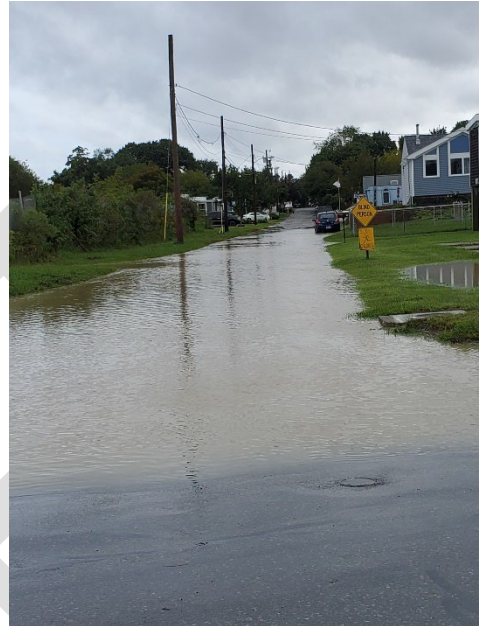
Flooding in Portsmouth.
