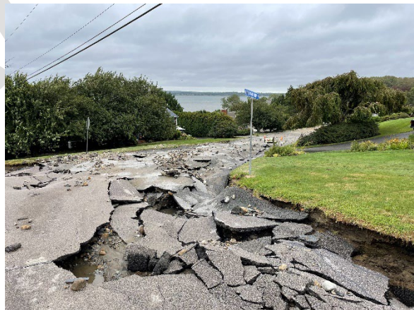
Road (above) and underground catch basin (left) collapsed after heavy rainfall from the remnants of Hurricane Ida in 2021.
