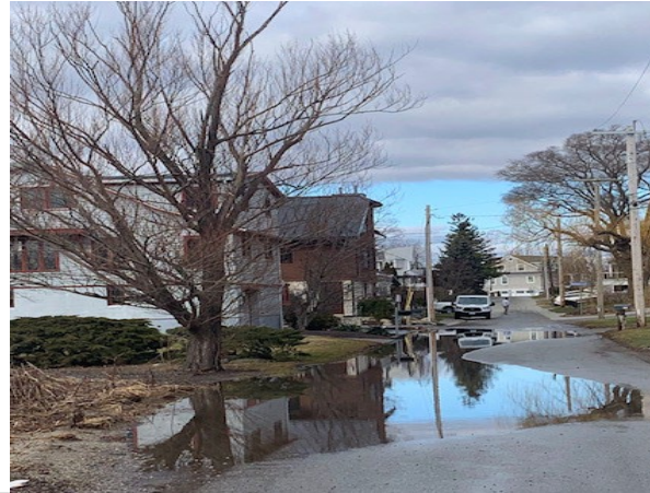
Flooding on Anthony Road, Portsmouth 2023.
